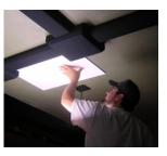
same three templates are used throughout to maintain uniform spacing. For flat ceilings, acoustic ceiling adhesive is used. Sloped ceilings will require additional
